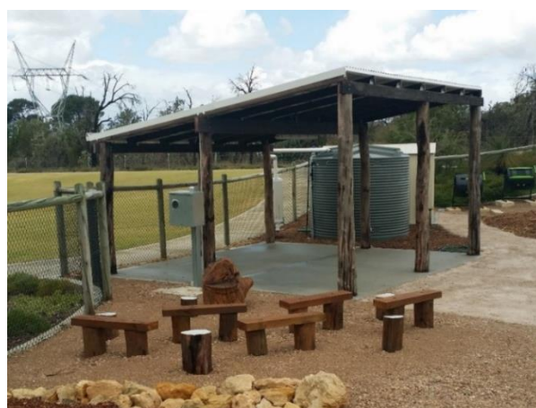
CCG covered shelter and outdoor classroom seating built from recycled and reclaimed timber. (Image supplied by Earthcare Landscaping)
