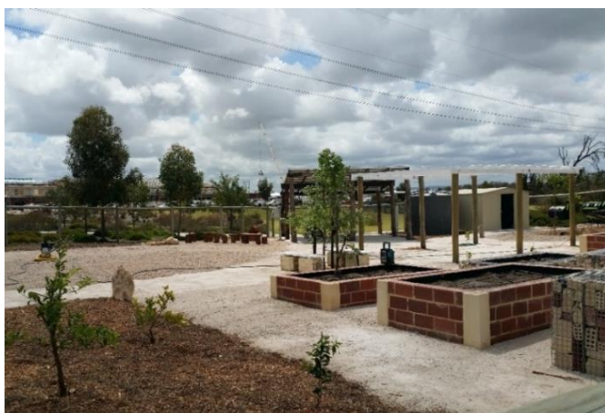
Recycled material used in the paths and recycled bricks used in planter boxes at the CCG. (Image supplied by Earthcare Landscaping)
